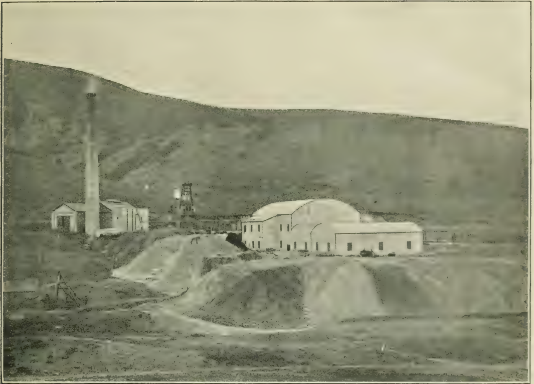
GLENCRIEFF SHAFT AND DRESSING PLANT OF THE WANLOCKHEAD COMPANY.
